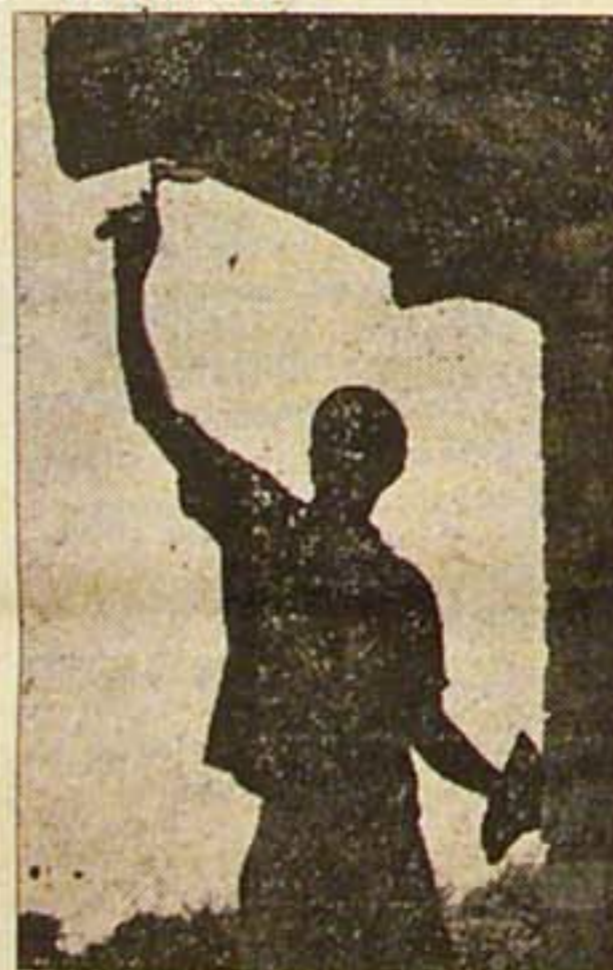
A house under construction in model Tanzanian village of Chamwino.
